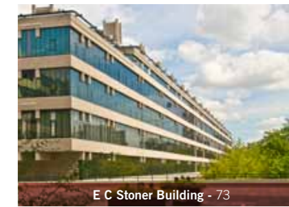
E C Stoner Building - 73
